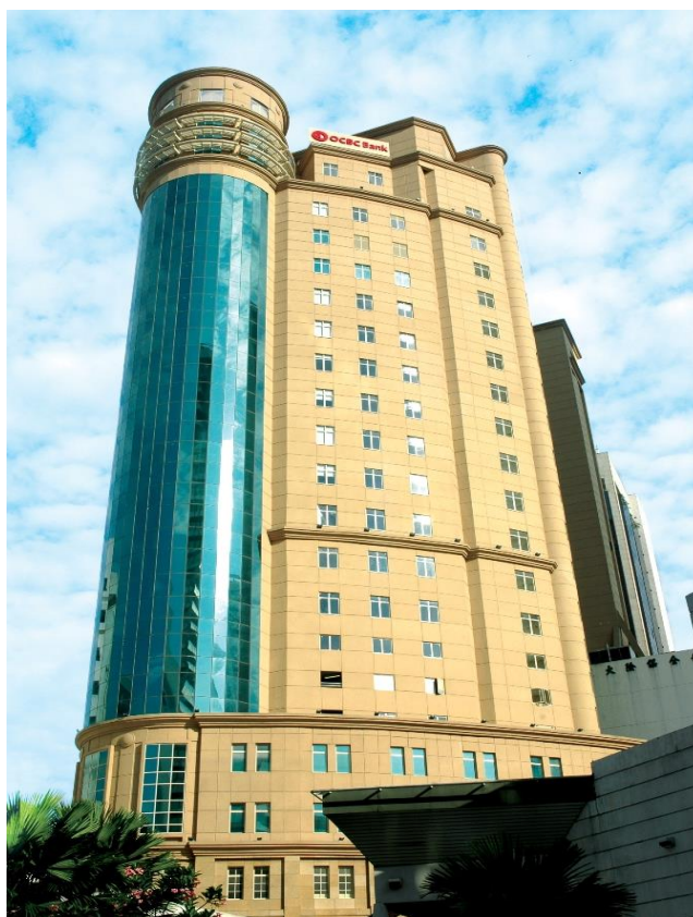
Menara OCBC, headquarters of OCBC Bank (Malaysia) Berhad
